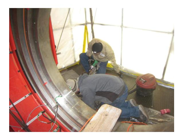
The 4 M12 through-holes for the support arm are drilled
